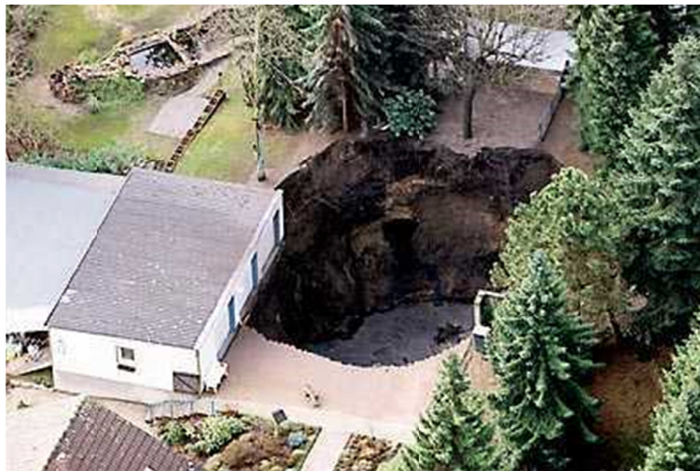
Fig. 4. Surface cave-in over an abandoned shaft
