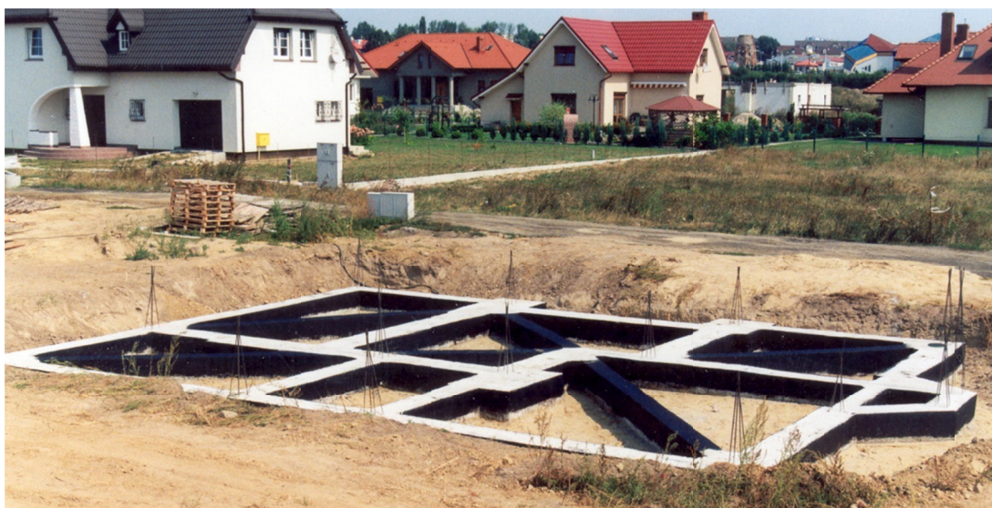
Fig. 1. Example of the use of diagonal braces at the foundation level
