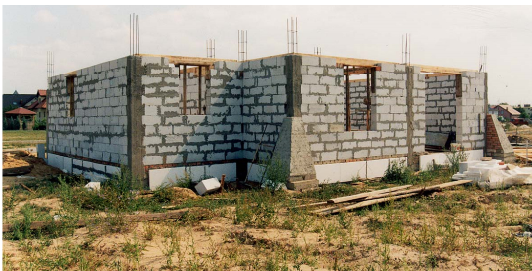
Fig. 2. Example of the use of reinforced concrete pillars in wall corners of a traditional building
